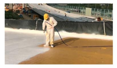
Project Contractor GCP Solutions Liantang Highway Chun Wo Construction Holdings Company Ltd ELIMINATOR<sup>®</sup> bridge deck waterproofing
