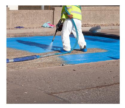
The transportation infrastructure design required a system that would offer a waterstop system – with water excluding and water retaining properties. This kept water within the canal and ensured that water could not penetrate the concrete tunnel.
