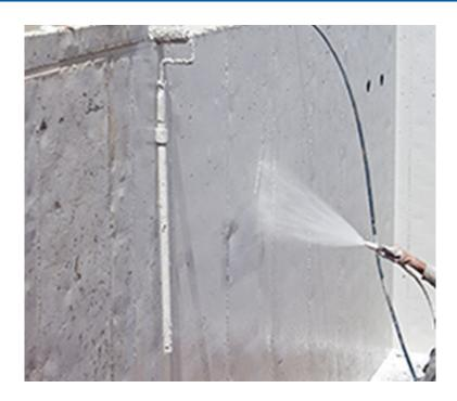
While bustling McCarran International has more than 1,300 slot machines located throughout its existing terminal buildings, the Department of Aviation wasn't gambling with the Terminal 3 airport construction. Because the train station and utility tunnel were in the water table, waterproofing was critical. The materials specified provided trouble-free resistance to hydrostatic pressure from the groundwater—and had to be installed during cold and severely hot weather.
