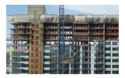
The high-rise contains two massive concrete cores with walls up to three-feet thick which were created using approximately 8,000 cubic yards of SCC and a new stateof-the-art admixture technology, ADVA <sup>®</sup>408.
